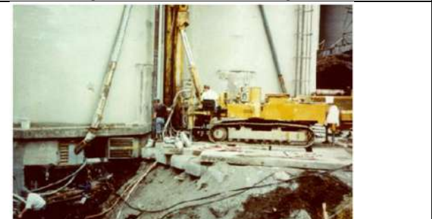
Fig. 4. Drill Rigs a) Large Track-Mounted Rotary Hydraulic Drill Rig
