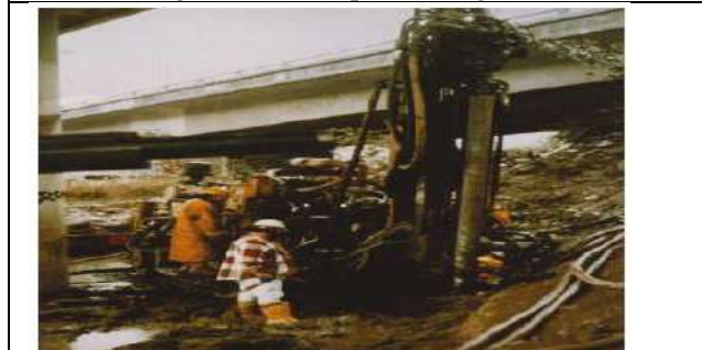
Fig. 3. Seismic Retrofit of I-110, North Connector, Los Angeles, California
