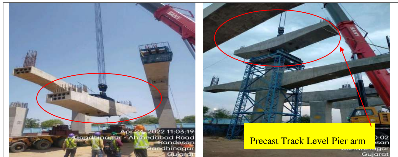
Fig.1. Station Cantilever Pier arm Erection
