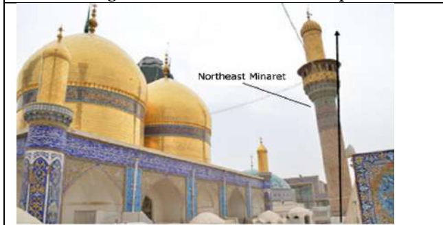
Fig. 7. Historical Minaret of Al-Kadhimin Mosque a) The leaning northeastern minaret
