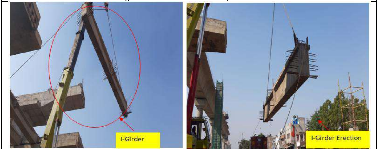
Fig-03. Viaduct & Station I-Girder Erection
