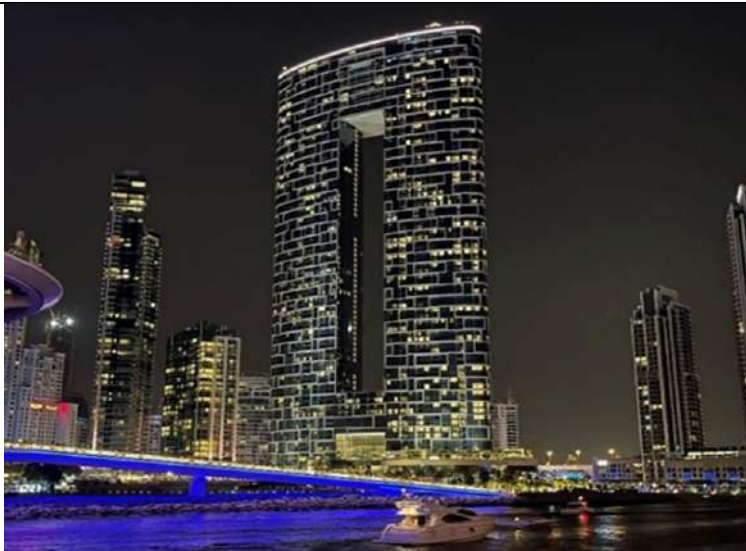
Figure 9 Twin tower (Source: -International journal of High-Rise Building) https://doi.org/10.21022/IJHRB.2022.11.1.61 [11]
