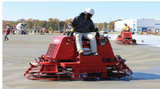
Fig. 4. Ride on power trowels
