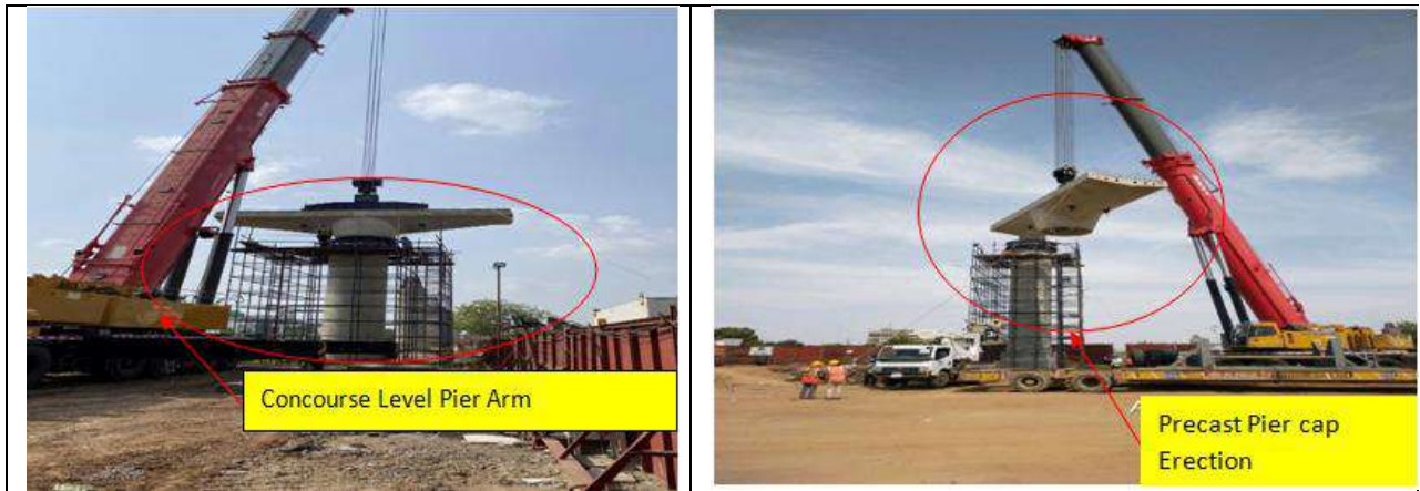
Fig-02. Viaduct Cantilever Pier cap Erection
