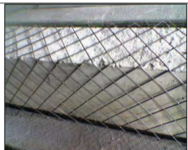
Fig.3.2: Orientation of Wire Mesh at 45 degrees
