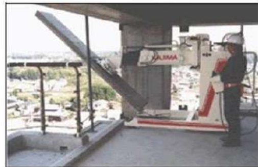
Fig 12. Wall installation robot in action by Kajima Corporation.
