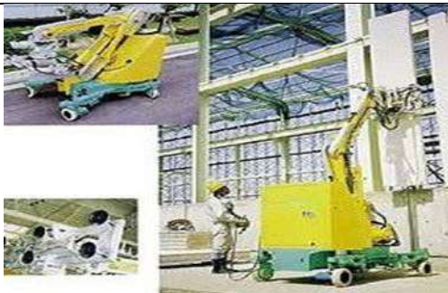
Fig 13. Multi-jointed handling robot for exterior material
