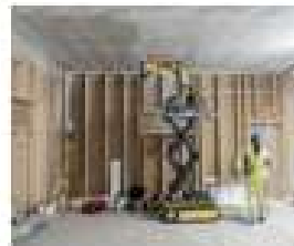
(g) Drilling robot
