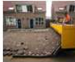
(c) Paving robot
